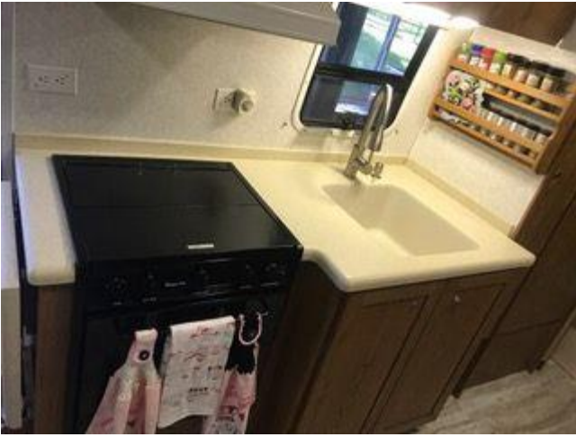
This is the new galley base with sink and stove installed.
