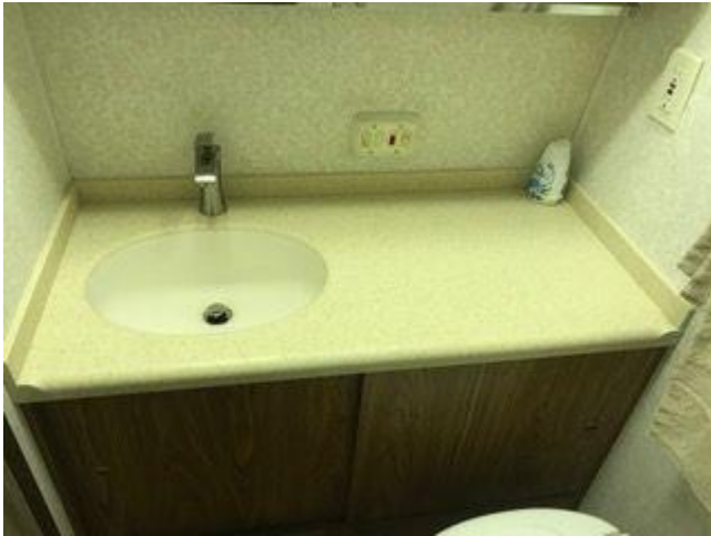
New vanity countertop and sink.
