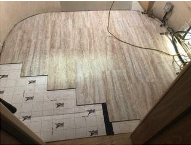
Starting the installation of the new flooring.
